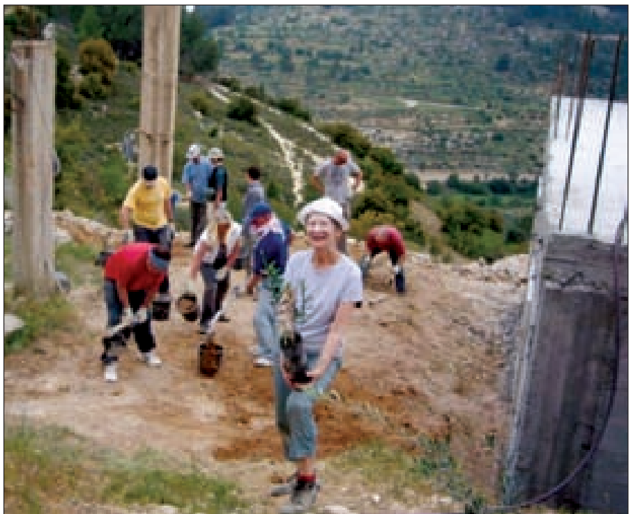
Anna in the foreground, with rebuilding team
